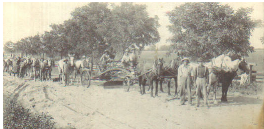
Borden Road west of Hubbardston
